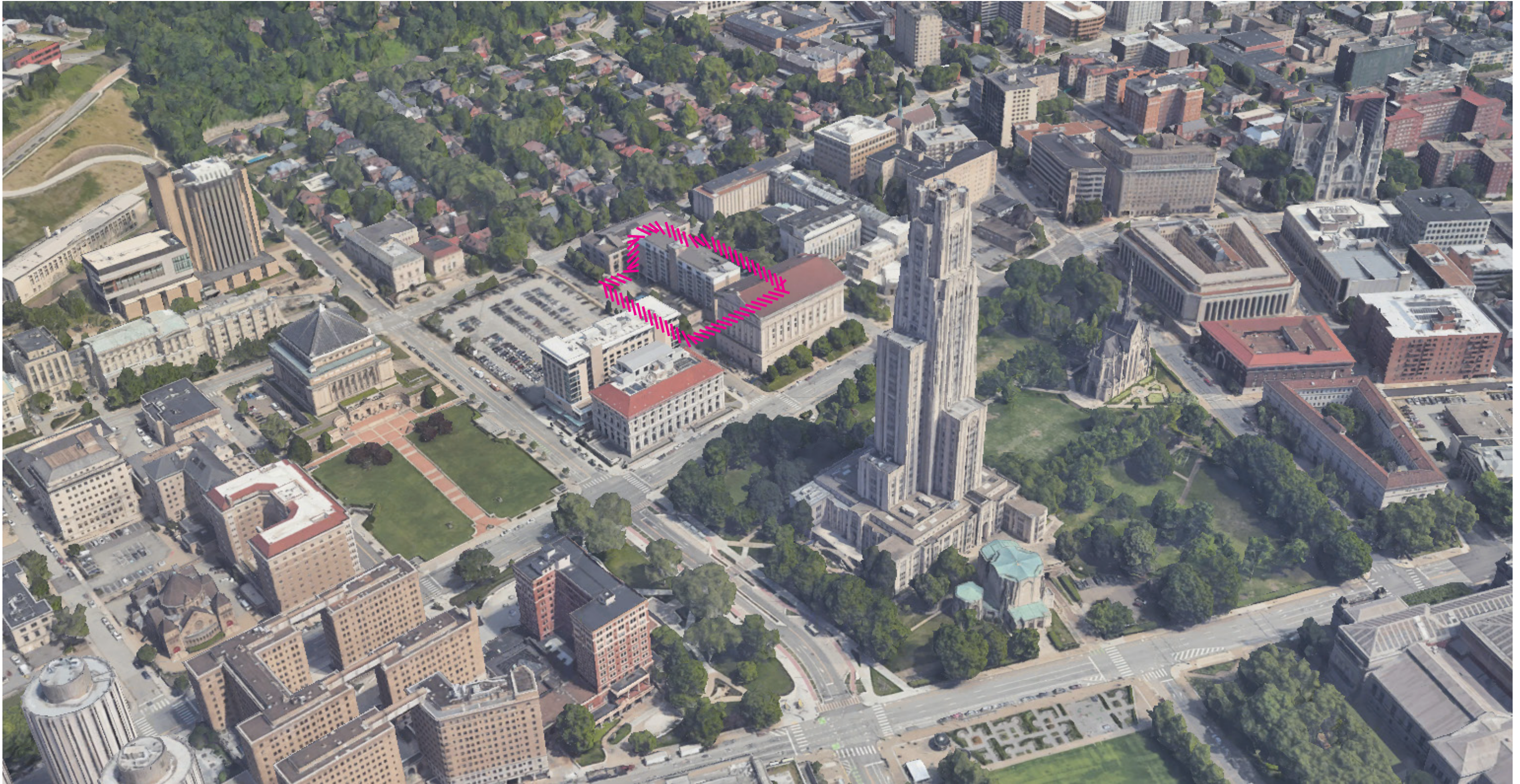
Aerial View to North with Cathedral of Learning in foreground
