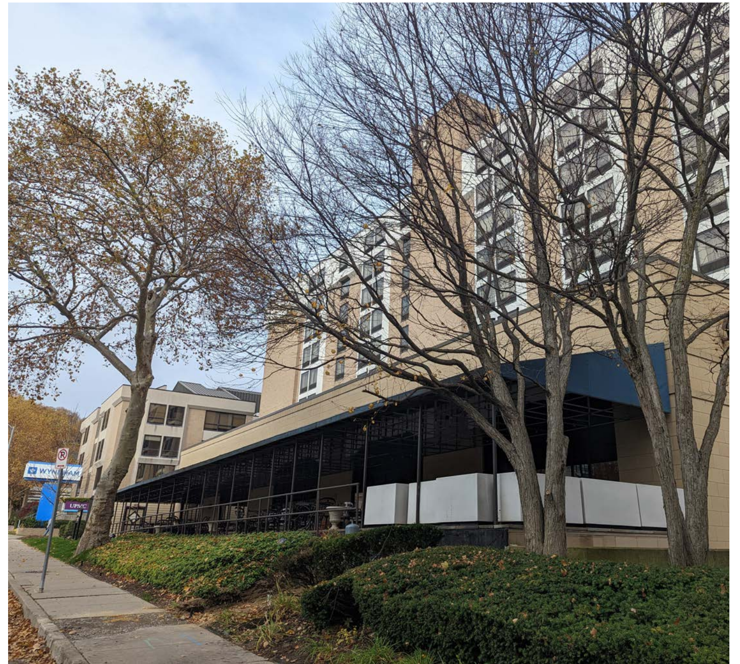
Photo 04 Patio Shade Structure
